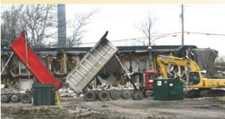
The demolition of the old Villager Inn was held up over the winter months due to permitting issues and asbestos removal. The property owner had to hire a new contractor to obtain the necessary permits and clear the site properly.
